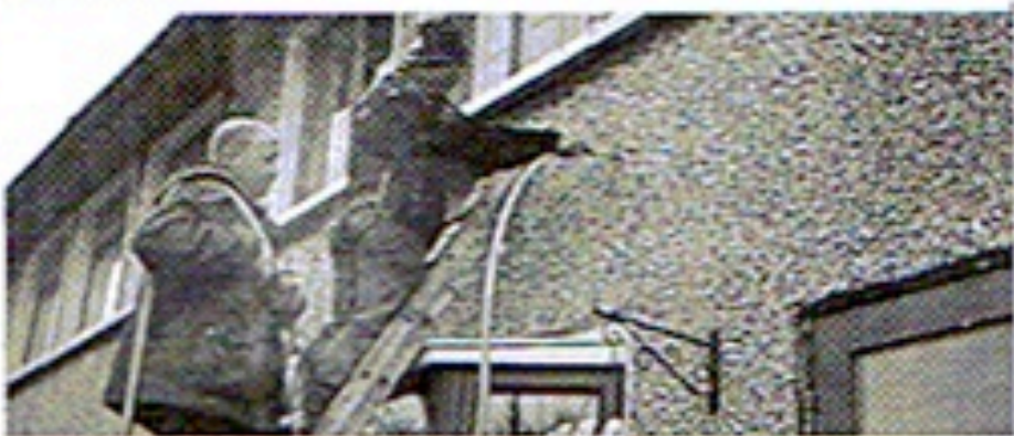
Picture shows the holes being filled with the foam.
